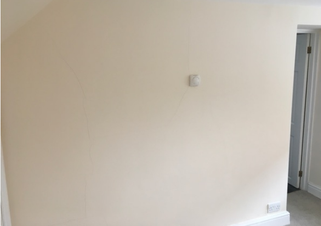
MOVE IN Cracking on wall
